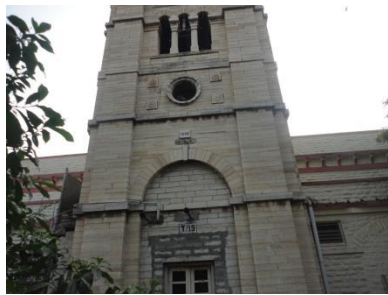
NEEMUCH RAILWAY STATION 1880
