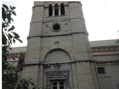
NEEMUCH RAILWAY STATION 1880
